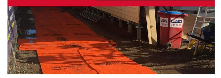
**Skudo All-Terrain Mat** provides an extremely durable, safe, slip-proof surface ideal for use on uneven, gravel or muddy construction sites. Bright, thick All-Terrain Mat indicates a designated pathway for workers, contractors and visitors, protecting them from hazards.
