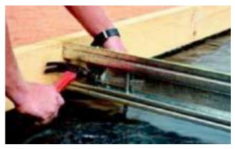
Adjust the keyjoint to the correct height and secure by tapping in the supplied wedges.
