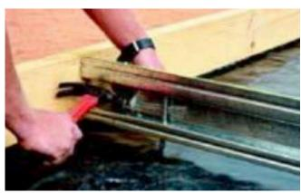
Place the reinforcement and pour the concrete over the keyjoint. Finish concrete surface to the top of the joint (NOT ABOVE IT). Always pour concrete evenly to both sides of the joint and ensure concrete is compacted into the keyways.
