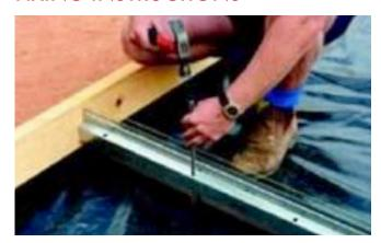
Position keyjoint in desired location and drive in the supplied pegs.
