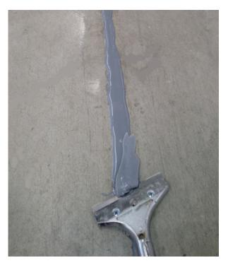
**HARDNESS:** The load support offered by both products is determined by their respective Shore A hardness. The higher the reading, the stiffer the filler. ACI and PCA call for a minimum hardness of A80. All Metzger/McGuire fillers exceed A80.
