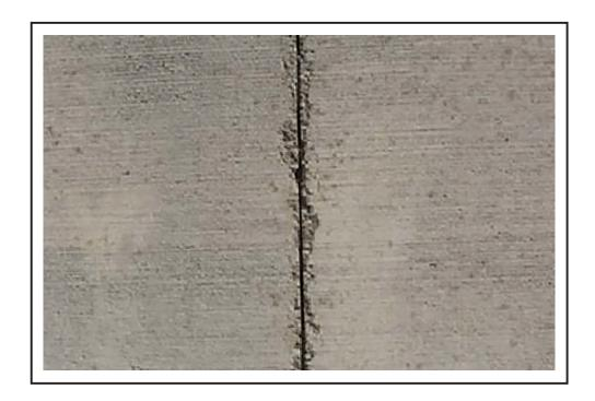
Joint deterioration is gradual but inevitable when an inferior filler is chosen or if a filler is installed poorly or no joint filler is installed at all. As the deterioration increases, the cost of repairs increase and your productivity decreases.
